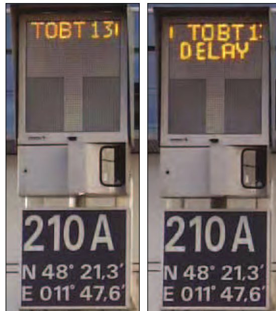
Large TOBT display in front of aircraft for Ground Handler staff and pilot awareness
